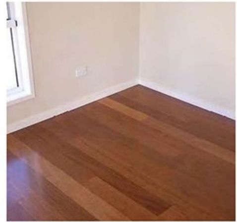
Site sanded and coated engineered floor
