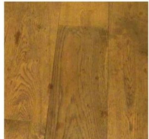
Oil finish – Severe staining due to insufficient care.
