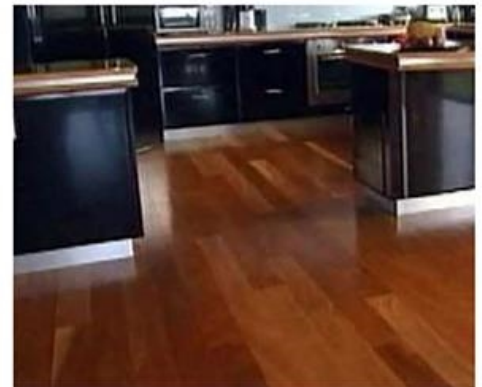
A completed site sanded and coated floor
