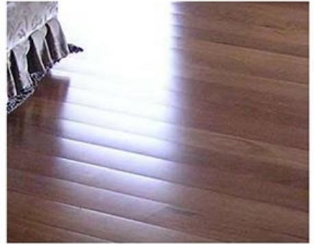
Higher humidity internal environments resulting in crowning
