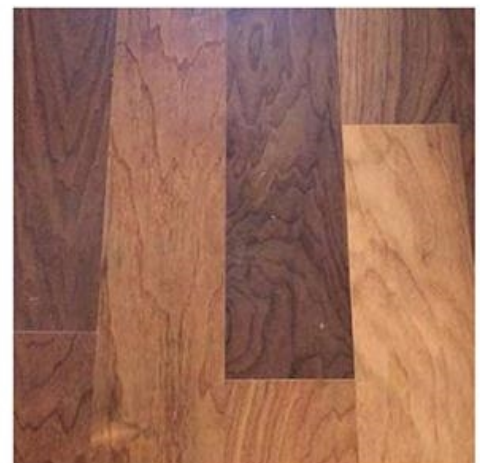
Boards are staggered so that ends do not cluster
