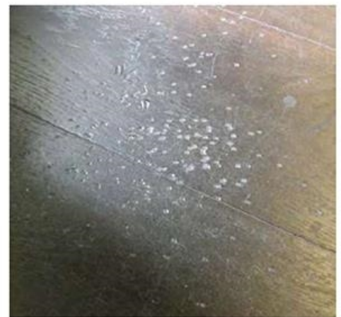
Oak is not a hard timber and in some high traffic commercial applications it can indent significantly.
