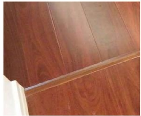
Control joint at the end of the hallway
