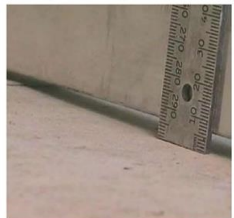
Subfloor flatness needs to be within the required tolerance
